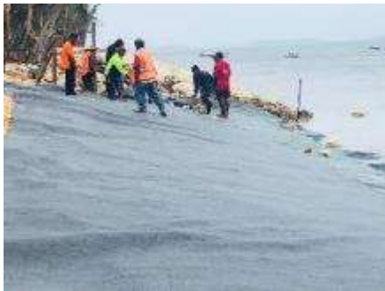
Figure 5 HCP geotextile work
