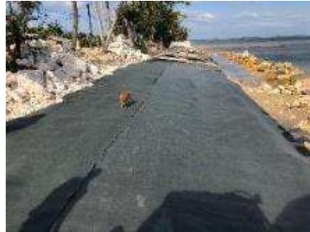
Figure 6 HCP geotextile work phase
